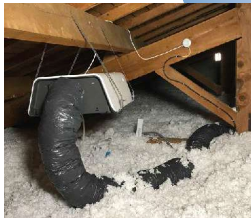
Pose comble VPS
